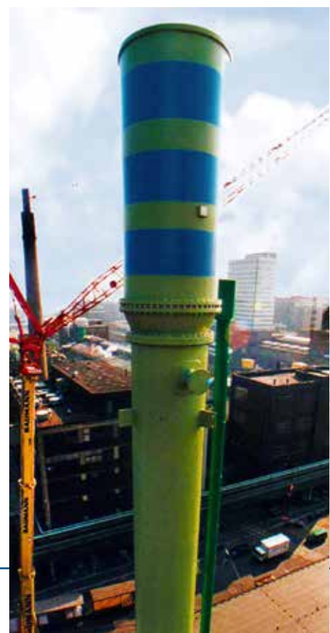
Körting droplet separator during transportation and installed on the chimney of a plant.
