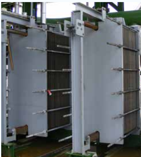
The closed loop water is re-cooled by clean cooling tower water in plate heat exchangers.
